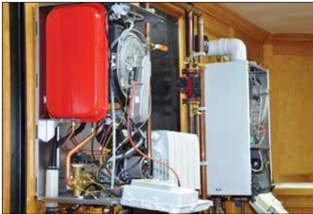
The gas-adaptive Baxi Luna Duo-Tec wall-hung boiler features removable front and side panels.
