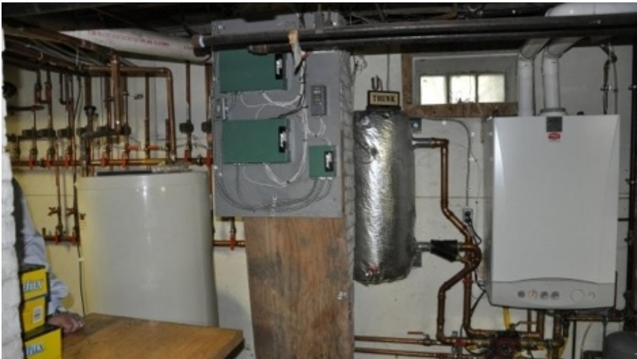
The mechanical room, with wall-hung boiler at right, thermal storage tank at left, and zone valve relays in the center.
